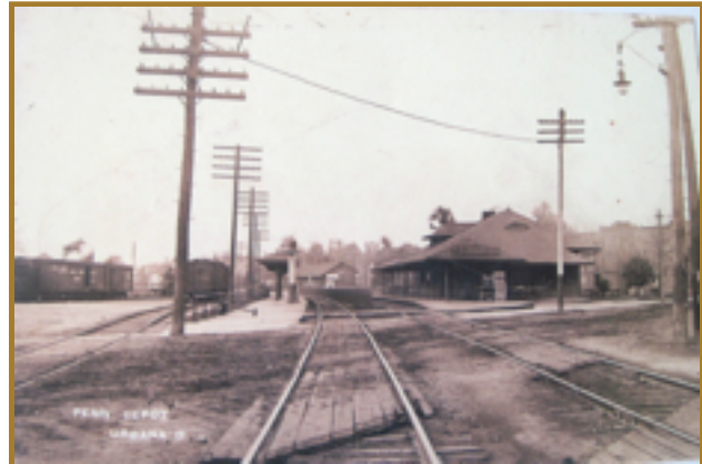
Urbana Depot as it looked back in the days when the PRR was running trains through Urbana to either Columbus or Indianapolis.
