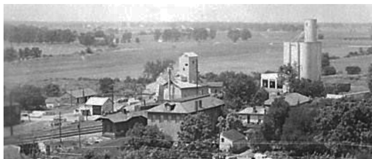
Figure 1 PRR Bradford Side Plain City with depot, factory, and grain elevator
